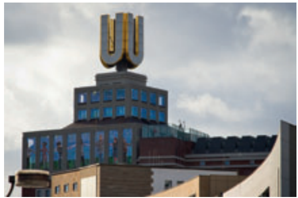
Figure 5.6-4 The ‘U-Tower’ in Dortmund. The former Union brewery has been converted into a creative centre – and become an emblem of the city. Source: Moellerh/Flickr
